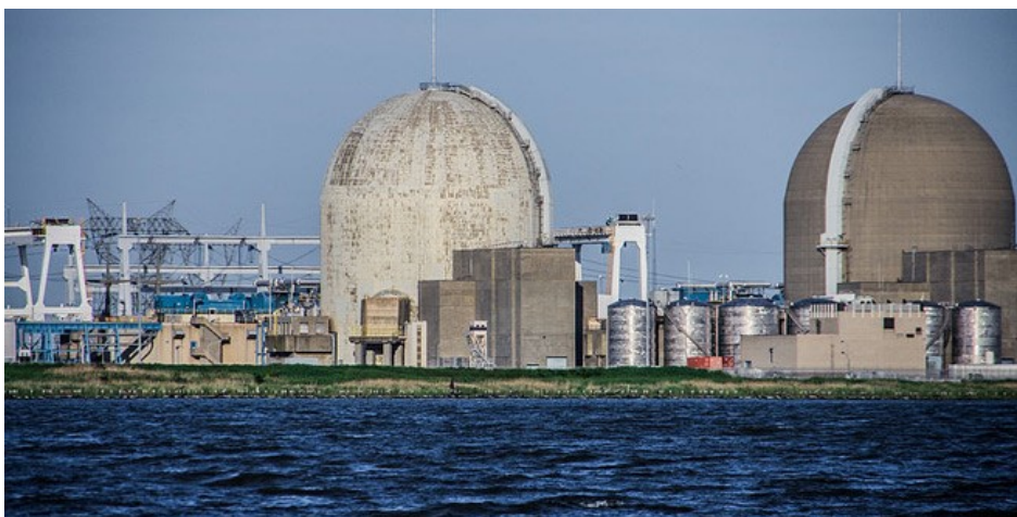
Salem nuclear plant on Artificial Island
